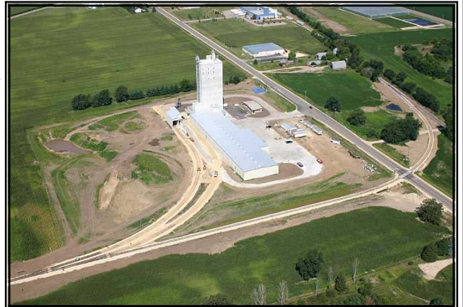
Cargill Animal Nutrition in Milton finishes construction on its rail spur located in the Milton Industrial Park.
